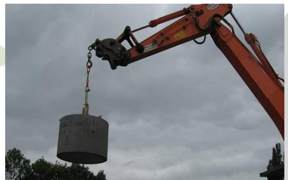
For the SVZ UNI lifter, adaptors are required to lift DN1800 chamber rings.
